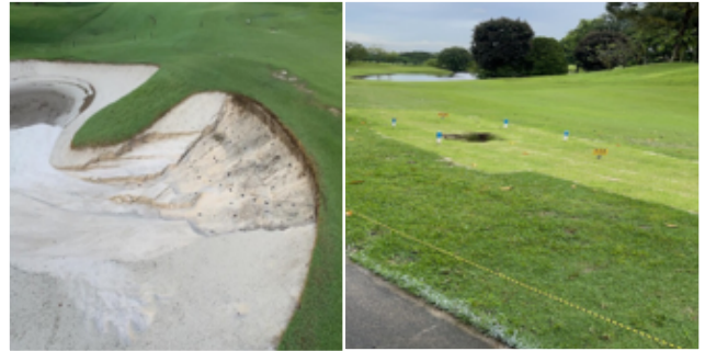
Collapsed faces of bunker and sunken holes caused by soil erosion
